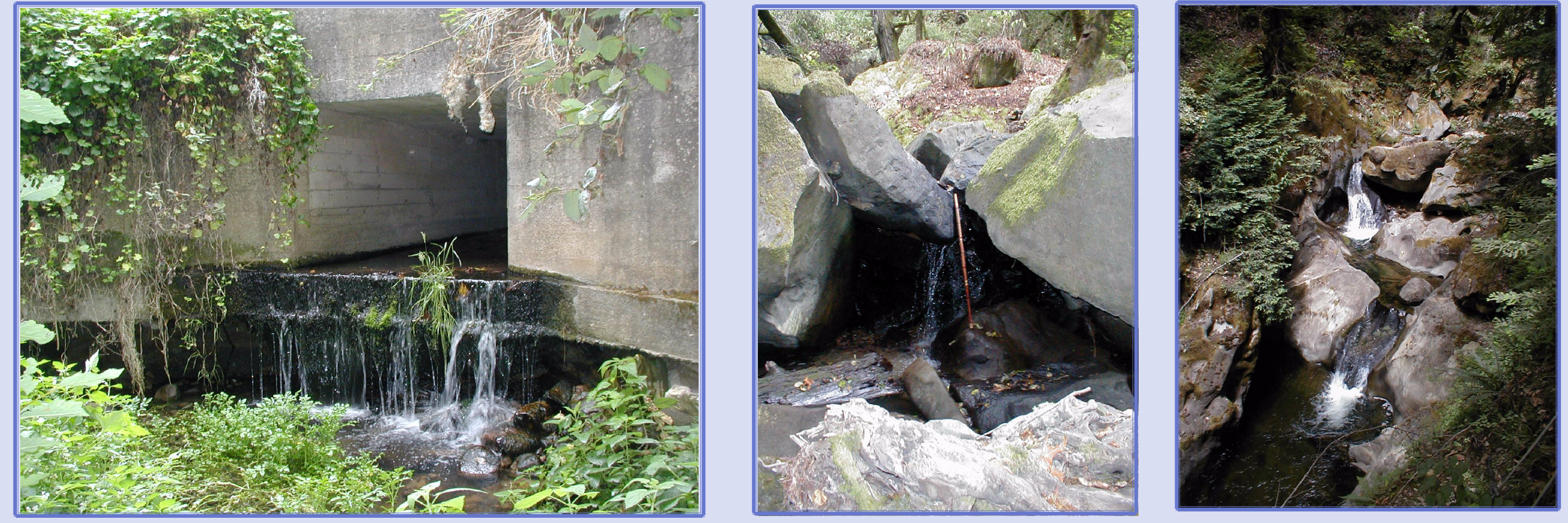
LI-5 - Perched Culvert on West Liddell Creek - Bonny Doon Road MA-1 - Boulder Cascade on Majors Creek SL-14 - Boulder Cascade on Kings Creek
